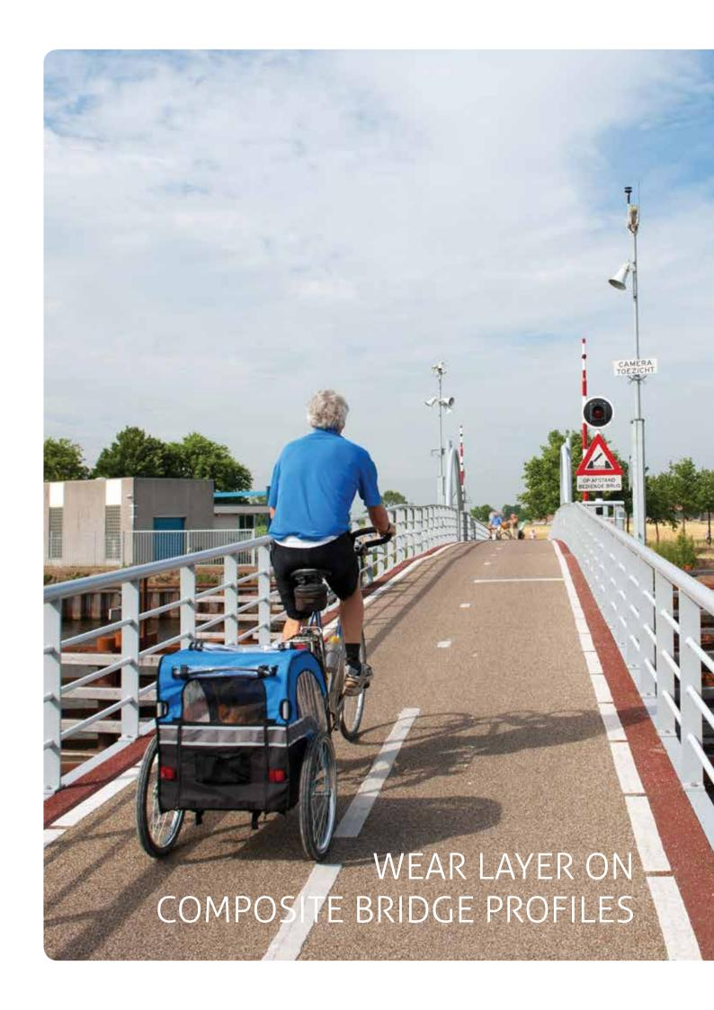
Over the last 10 years, the demand for bridges made from composite profiles has increased significantly. That is due to the relatively low weight, the durability and low maintenance costs of such profiles. The unique supporting structures consist of pultruded, glass fiber reinforced polyester profiles and the girders are in composite. For the bridge surface, composite bridge deck boards are used. These must be provided with a trafficable wear layer.
