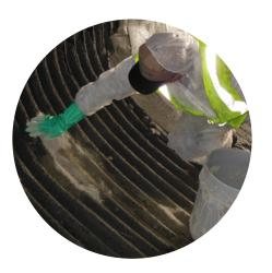
All active water leaks and infiltration is plugged and patched with Custom Plug® hydraulic cement. Chemical grout injection or flowable fill grout pumping may be used for filling large voids around pipe.
