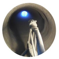
Depending on the pipe size and configurations, use either the GeoCast™ Pipe Renewal spin-cast head and sled or a low pressure, air atomising, wet shotcrete nozzle for applying a monolithic, geopolymer liner.
