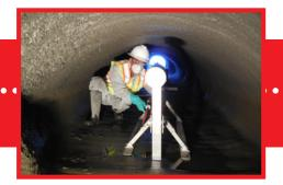
As a **Sustainable Green Technology** the GeoCast<sup>™</sup> Pipe Renewal system uses a patented spin-cast geopolymer lining technology. This high performance, fibre reinforced, corrosion resistant mortar is placed by centrifugally casting or using an air atomising shotcrete nozzle to apply the geopolymer liner.
