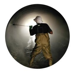
Pre-installation cleaning and inspection is performed to identify pipe material, pipe size, pipe length and defects. High pressure water blast at minimum 4000psi is required for adequate removal of rust, dirt and laitance.
