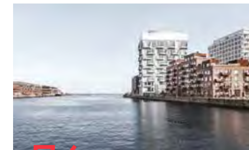
74 Silo in Copenhagen Microtopping®
